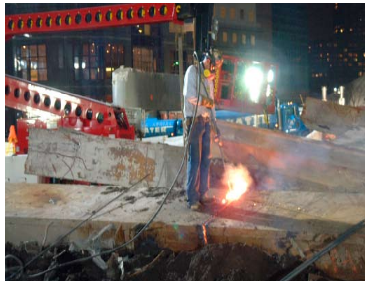
Cutting Down Structural I-Beams for Hauling
